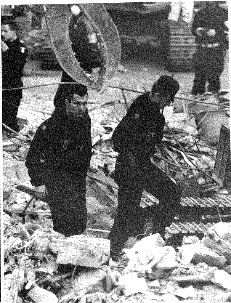
French rescuers inspect the debris of a building KYODO
